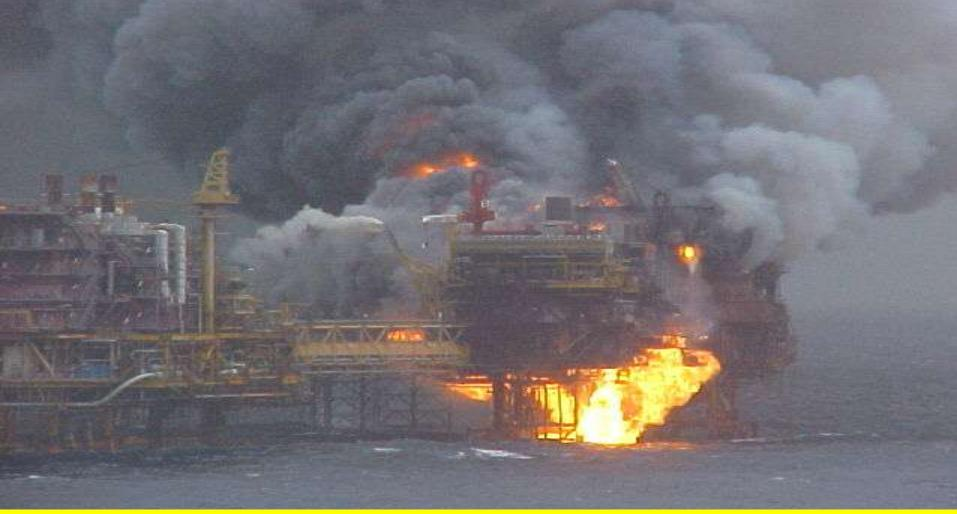
On 28 July 2005 the dive support vessel collided with the installation, the edge of the vessel's heli-deck cut the pipe. 10 employees (from 220) and 40% of India's crude oil supply were lost.
