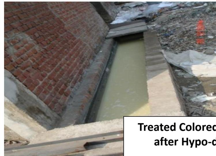
Treated Colored Effluent after Hypo-dosing
